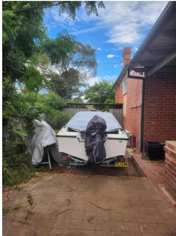
Rear view of existing carport area, to replaced with new, longer carport
