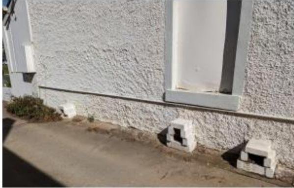
8. Previous treatments using ventilation of the sub-floor.
