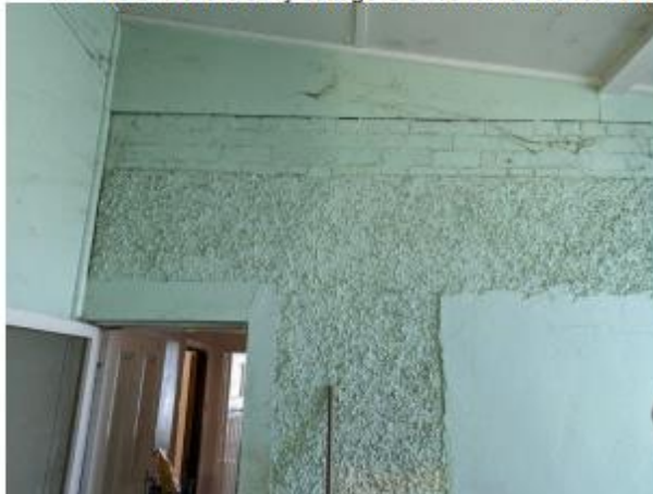
18. A portion of the rendered wall and the door to the main passage. The wall is in a roughcast finish plus the extra brick courses over to allow for raising of the roof
