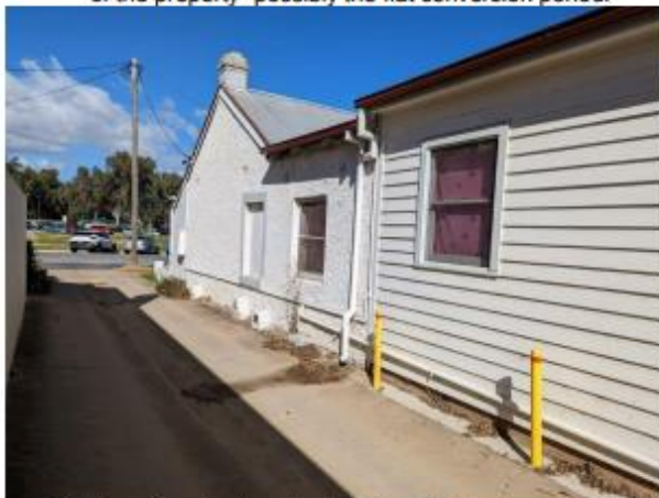
10. View from the Lane looking towards the frontage showing the original and extension elements. Windows if retained on the boundary wall will need treating to meet the BCA conditions.
