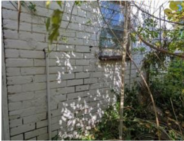
9. The later stretcher bonded brick to the rear laundry/toilet block indicates this is a later stage of the property -possibly the flat conversion period.
