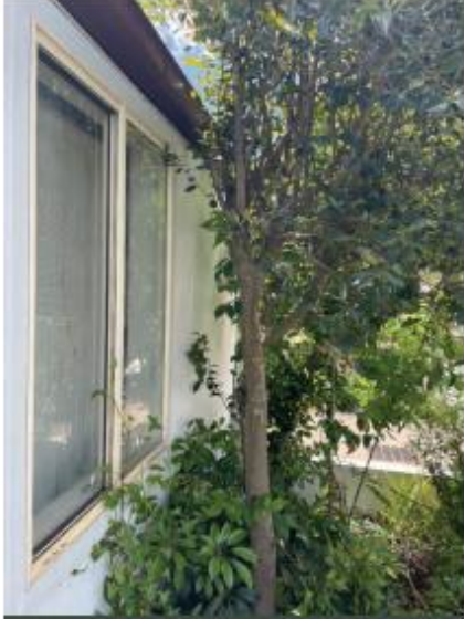
Privet trees growing too close to building need to be removed. Will cause structural damage
