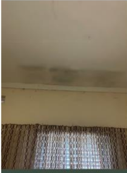
Mould to ceiling
