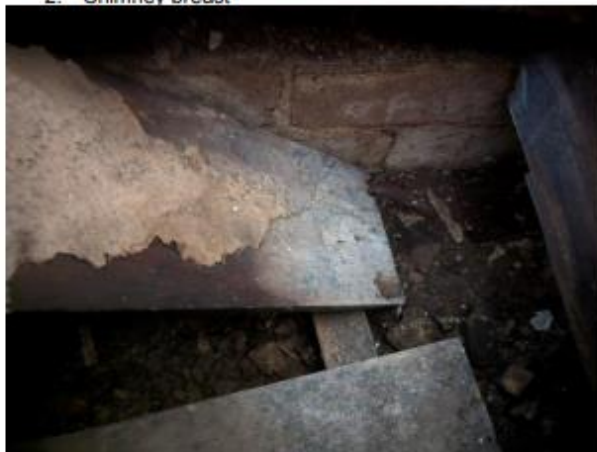
3. View into minimal sub-floor area. Engineering advice will determine whether this can be conserved as a ventilated sub-floor with steel joist construction or a concrete slab replacement installed.
