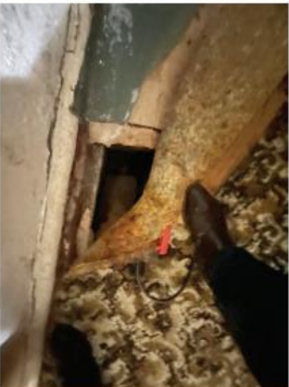
Rotten flooring in the lounge room. Sub floor is approximately 200mm below floor height and is saturated with ground water.
