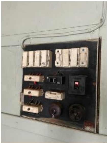
EDB without earth leakage protection
