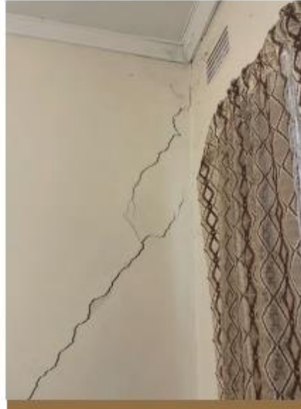
Internal structural cracking to bedroom
