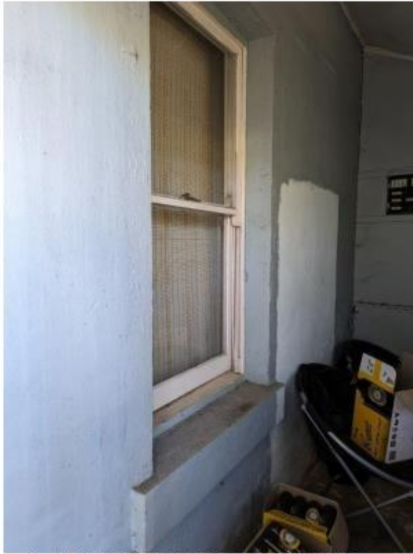
6. A replacement DHSS with rendered wall and sill
