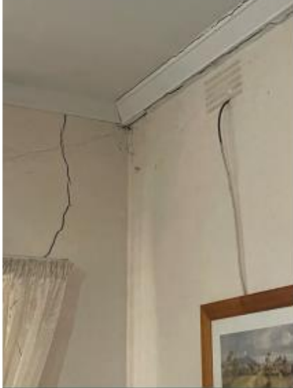
Structural cracking to the lounge room
