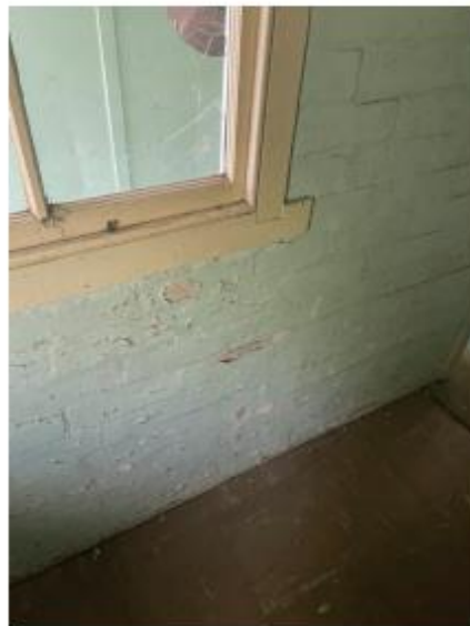
Peeling paint to rear room, probably contains lead
