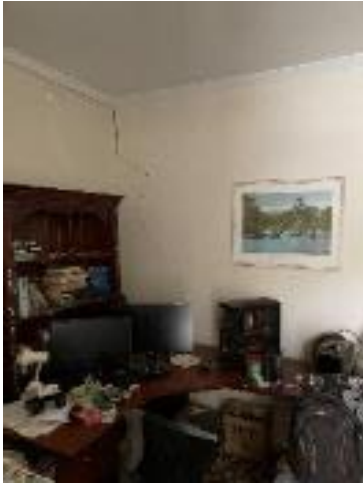
Cottage - front living room cracking
