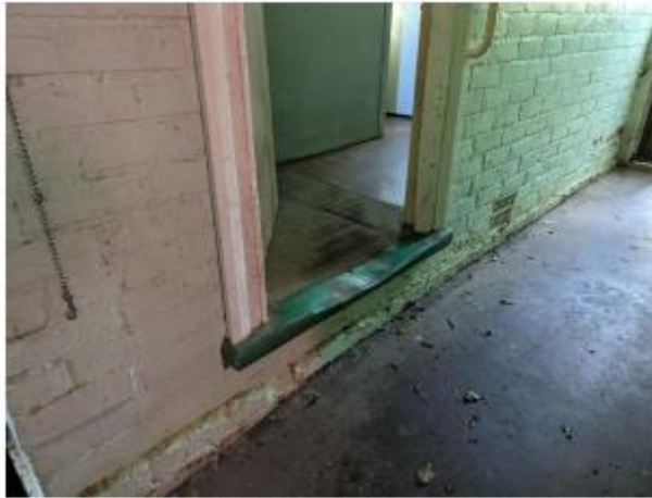
17. The end of the early cottage is evident with the rear threshold and brickwork
