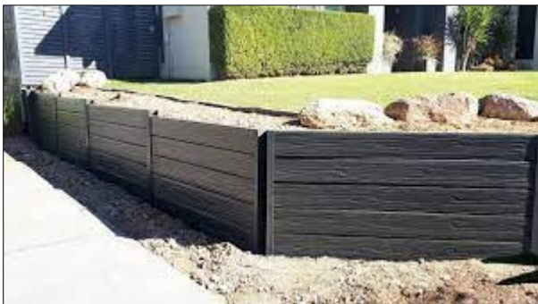
Figure 2 Example of concrete sleeper retaining wall
